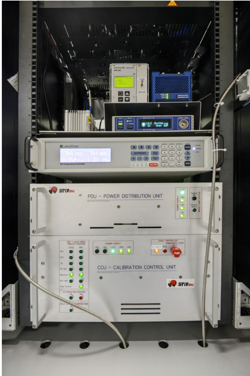
Figure 4. Electronic stages of the Calibration Unit.
