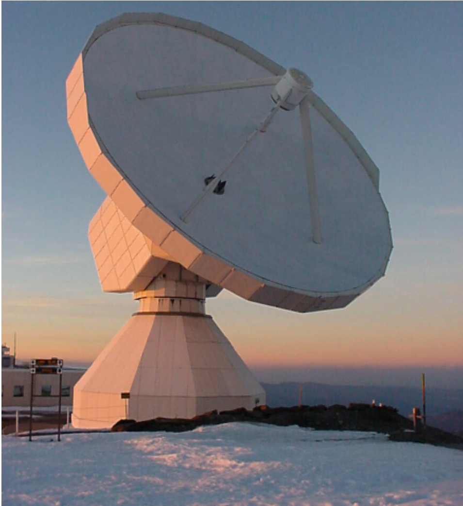
IRAM 30m telescope (Pico Veleta, Spain), altitude 2900m, surface accuracy 50 \mu\text{m}
